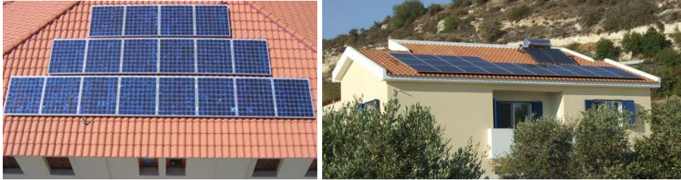
FIGURE 3: A 2.97kWp (LEFT) AND 4.2kWp (RIGHT) PV SYSTEM INSTALLATIONS
